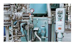
In the Toa Oil FCC Plant in **Japan** the Sundyne API 610 type OH6 reactor recycle pump handling Butane is operating successfully with a dual pressurized face-to-back EagleBurgmann API 682 type A pusher seal. It runs with plans 13/54 at 20.000 min<sup>-1</sup> at a sealing pressure of over 66 bar (957 PSI).
