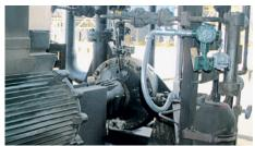
To convey sour water with high SO<sub>2</sub> content, a Weir pump is installed in the fluid catalytic cracker (FCC) of the Amuay-Cardón refinery in Venezuela. The shaft is sealed by dual pressurized EagleBurgmann API type A seals and equipped with a barrier fluid system with bladder accumulator. Configuration 3CW-BB, piping plans 02 and 53B. Operating conditions: p = 15 bar (218 PSI),  $t = 50 \, ^{\circ}\text{C} (122 \, ^{\circ}\text{F}), \, n = 3,600 \, \text{min}^{-1}.$
