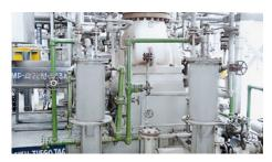
A dual EagleBurgmann API type C double ply bellows seal performs well in a Kirloskar Ebara debutanizer reboiler pump which is installed in the RPL refinery complex in Jamnagar, **India**. Configuration: 2CW-CW, piping plans 21, 52. Shaft diameter: 130 mm (5.12"). Operating conditions:
