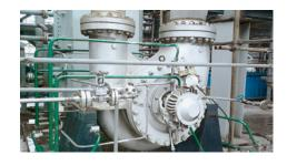
Fujian Refining & Petrochemical Co., Ltd. in **China** applies a BB2 pump for propane de-asphalting. The shaft seal is an EagleBurgmann API type A seal. Configuration 2CW-CW, piping plans 21+52. Operating conditions: p=73 barg (1,059 PSIG), t=165 °C (329 °F), n=2,970 min<sup>-1</sup>.
