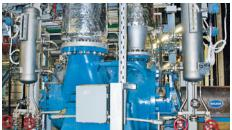
Since commissioning in January 2009, one of the critical pumps in the Bangchak refinery, Bangkok, **Thailand** performes well with a dual EagleBurgmann API type C metal bellows seal with an unpressurized buffer fluid system. Configuration: 2CW-CW, pipings plans 23, 52. Operating conditions:
