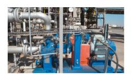
De-ethanizer pump in a LPG fractionation unit of ENOC refinery, **U.A.E.** equipped with an unpressurized dual EagleBurgmann sealing system acc. to API 682. Configuration: 2CW-CS, piping plans 14 and 76. Operating conditions:
