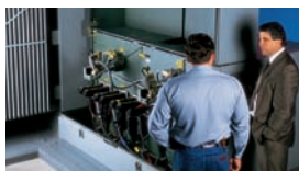
COOPER Power Systems
